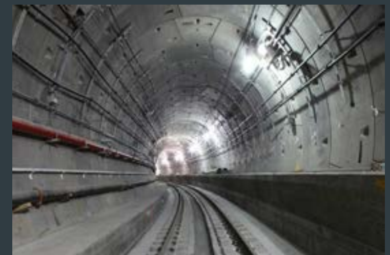
NEW YORK NO. 7 SUBWAY LINE
